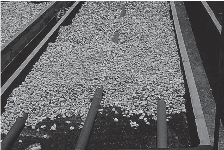
FIGURE 13.8 Drain-fill lines in bottom of beds. (From Hidroponias Venezolanas, S.A., Caracas, Venezuela. With permission.)
