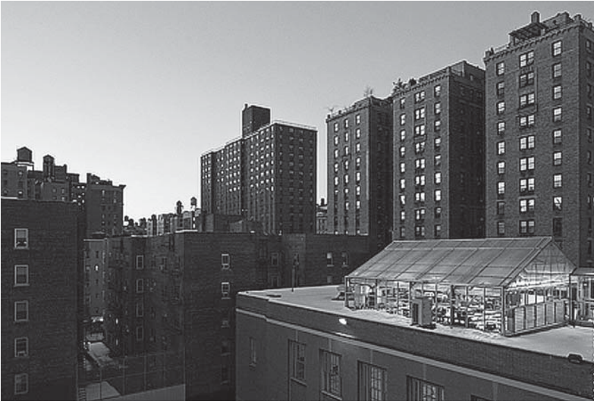
FIGURE 13.49 Rooftop hydroponic greenhouse at the Manhattan School for Children. (From New York Sun Works, New York, NY. With permission.)
