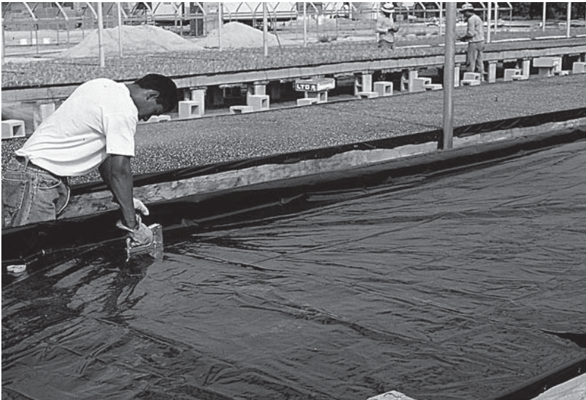
FIGURE 12.3 Black polyethylene liner is stapled to the bed. (From California Watercress, Inc., Fillmore, CA. With permission.)
