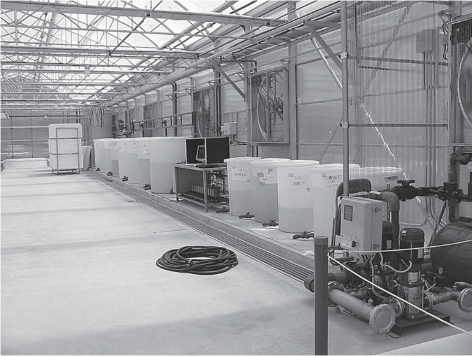
FIGURE 5.34 Adjustment of the nutrient solution using an injection system. (From Hydrinov, Inc., Japan Plantation Co. Ltd.-Nippon-Noen, Hiroshima, Japan. With permission.)
