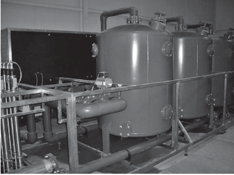
FIGURE 3.14 Filters on the right with UV on the left. (From Eurofresh Farms, Wilcox, AZ. With permission.)
