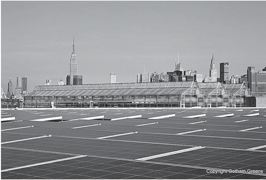
FIGURE 13.37 Gotham Greens greenhouse with solar array. (From Ari Burling & Gotham Greens, Brooklyn, NY. With permission.)
