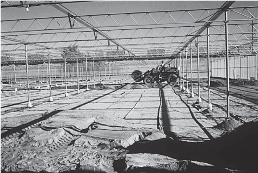
FIGURE 8.4 Back filling with 12 in. of sand.
