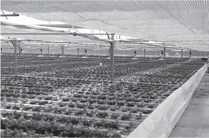
FIGURE 6.19 Perimeter polyethylene curtain around beds contains cooled air under the beds. (From F.W. Armstrong Ranch, Oak View, CA. With permission.)
