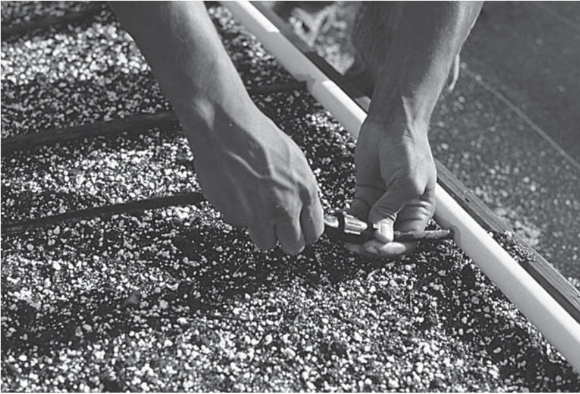
FIGURE 8.10 Attaching T-tape drip line to polytube adapter. (From California Watercress, Inc., Fillmore, CA. With permission.)
