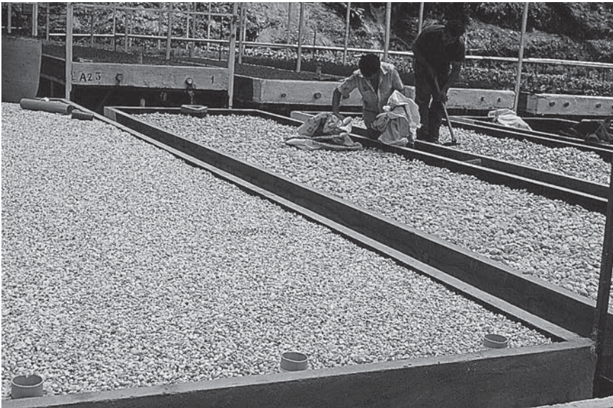
FIGURE 13.13 Coarse rock with pea gravel and finally a top layer of coarse sand. (From Hidroponias Venezolanas, S.A., Caracas, Venezuela. With permission.)
