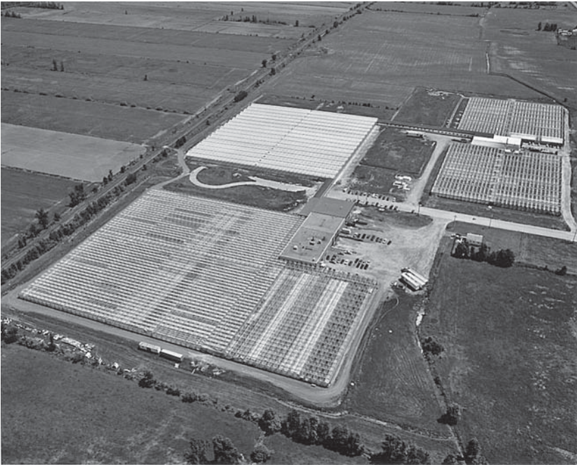
FIGURE 5.16 Hydroserre Mirabel, Inc., Mirabel, Quebec, Canada. (From Hydronov, Inc. With permission.)
