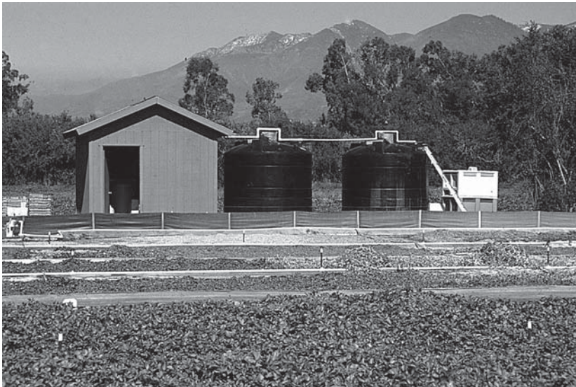
FIGURE 6.57 Two 2,300-gal stock solution tanks with injector shed on left. (From California Watercress, Inc., Fillmore, CA. With permission.)
