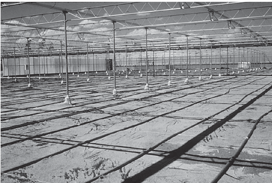
FIGURE 8.3 The laying of a polyethylene liner and drain pipes.
