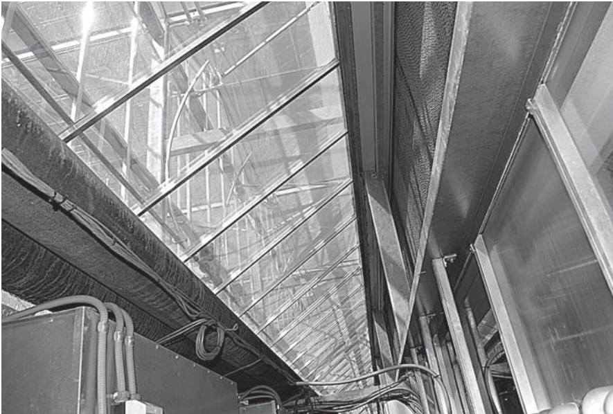
FIGURE 11.12 Evaporative cooling pad above on the right, glass shutter directly above. Note: The shutter is fully open for cooling cycle. Hot water mains on the left. (From Houweling Nurseries Oxnard, Inc., Camarillo, CA. With permission.)
