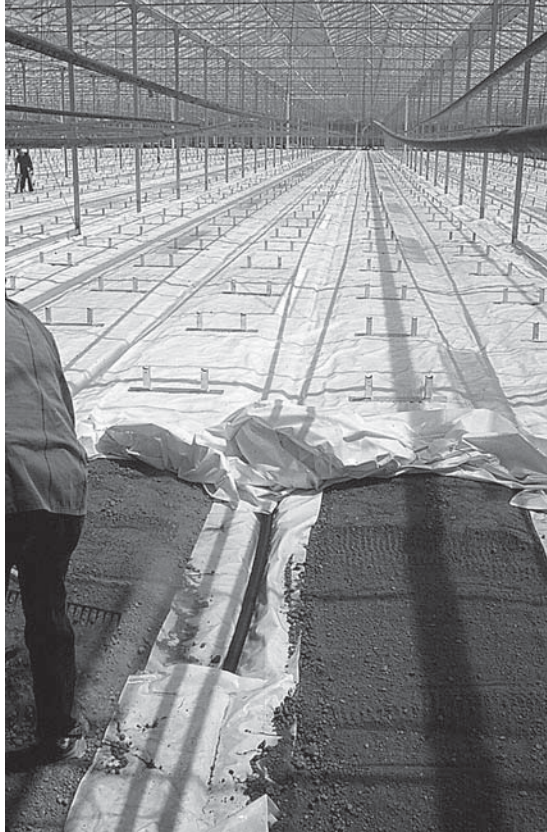
FIGURE 9.11 White-on-black polyethylene floor barrier. Note: The drainage pipe under the polyethylene floor barrier located in what will be the middle of the plant rows. (From Houweling Nurseries Oxnard, Inc., Camarillo, CA. With permission.)
