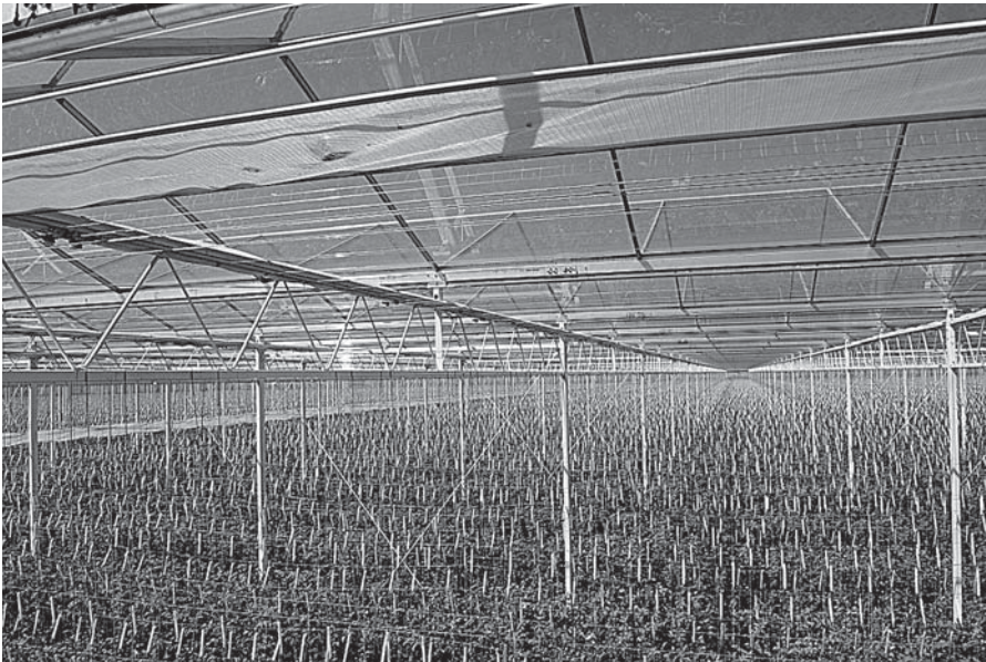
FIGURE 11.9 Powder coated structural membranes to improve light. Note: The height of the structure at the gutters is well above the crop. (From Houweling Nurseries Oxnard, Inc., Camarillo, CA. With permission.)
