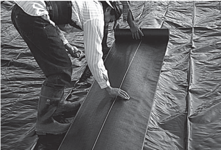
FIGURE 6.53 Cover berms with a 2-ft-wide nursery mat to prevent the sun from damaging the black polyethylene. (From California Watercress, Inc., Fillmore, CA. With permission.)
