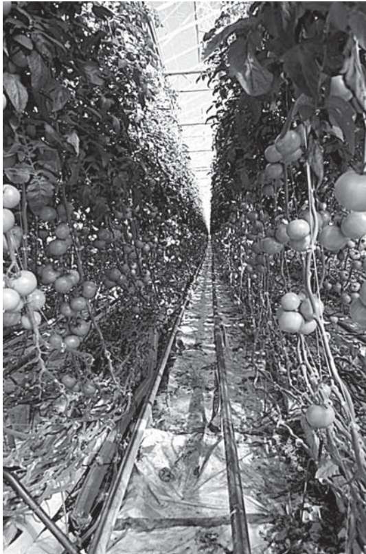
FIGURE 9.4 Sawdust culture with hot water heating pipes and carbon dioxide tube next to left pipe. (From Gipaanda Greenhouses Ltd., Delta, B.C., Canada. With permission.)
