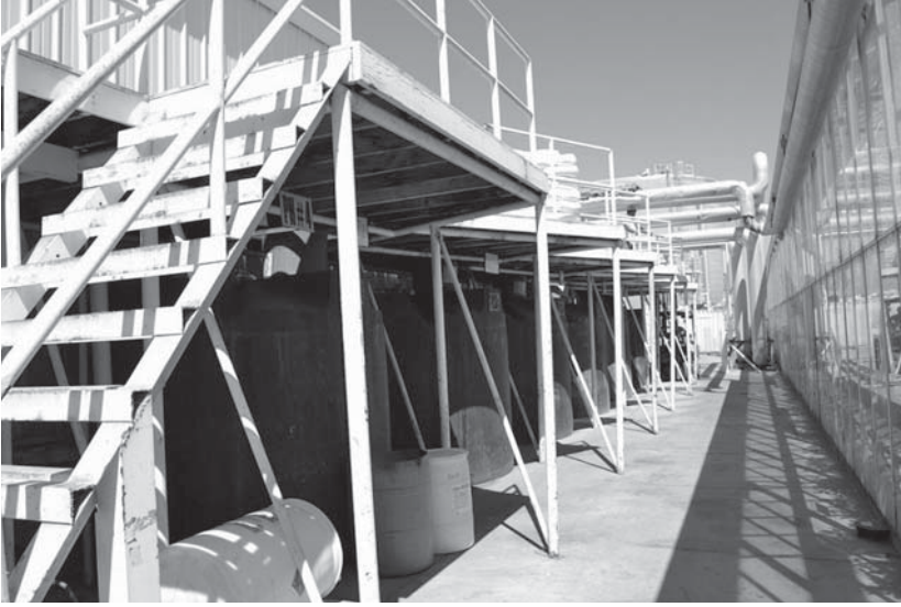
FIGURE 3.12 Stock tanks of 3,000 gal. (From Houweling Nurseries, Inc., Oxnard, CA. With permission.)
